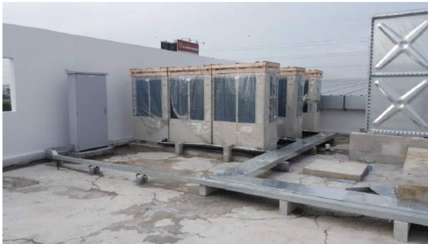
VRV System Final Positioning & Installation
