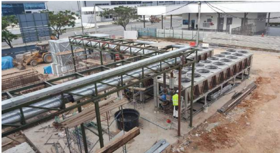
Chiller & Chilled Water Pipe Rack Installation
