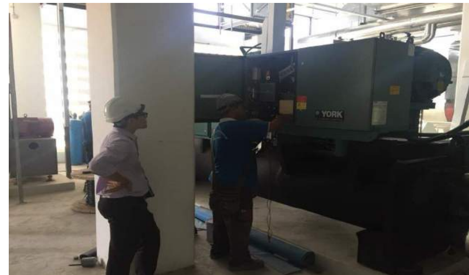
Chiller Final Electrical Connection
