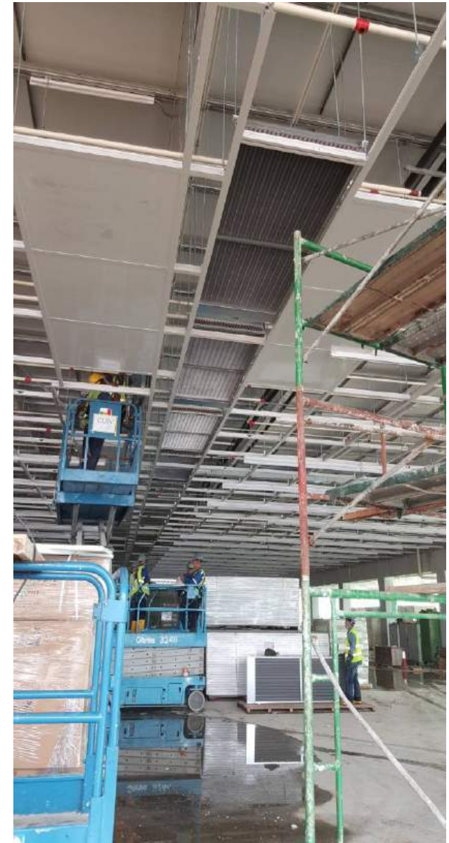
Dry Cooling Coil Installation #2
