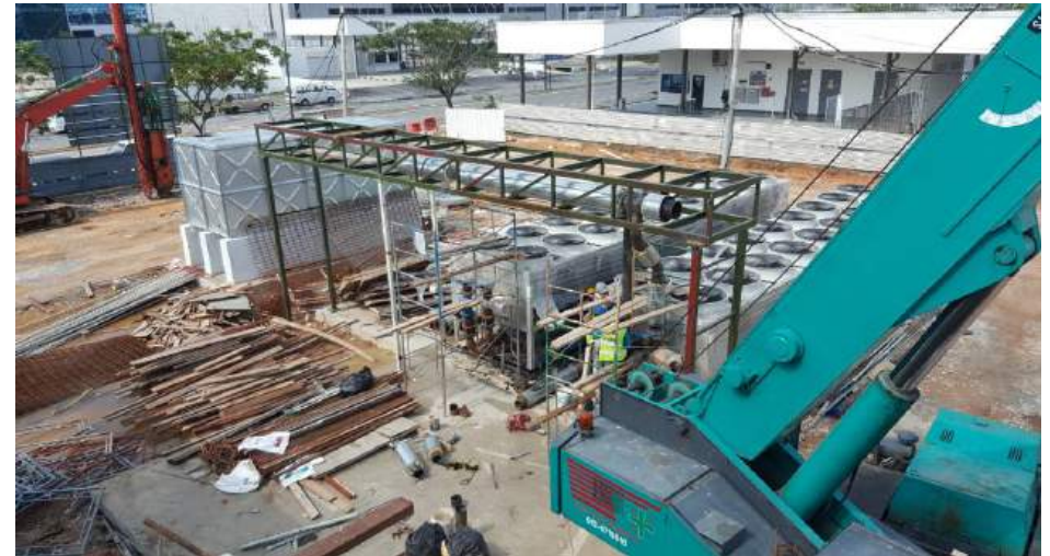
Chiller Final Positioning
