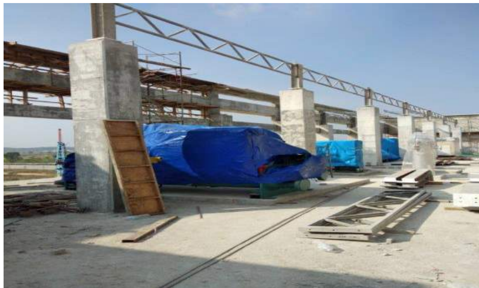
Chiller Moving In
