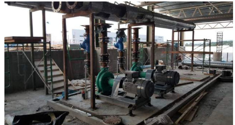
Chilled Water Pump Installation
