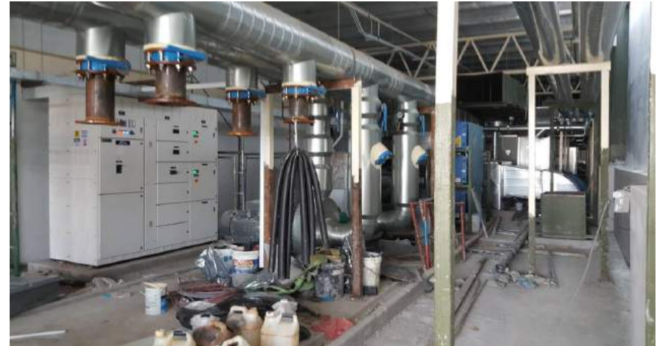
Plant Room MCC, Chilled Water Piping Installation
