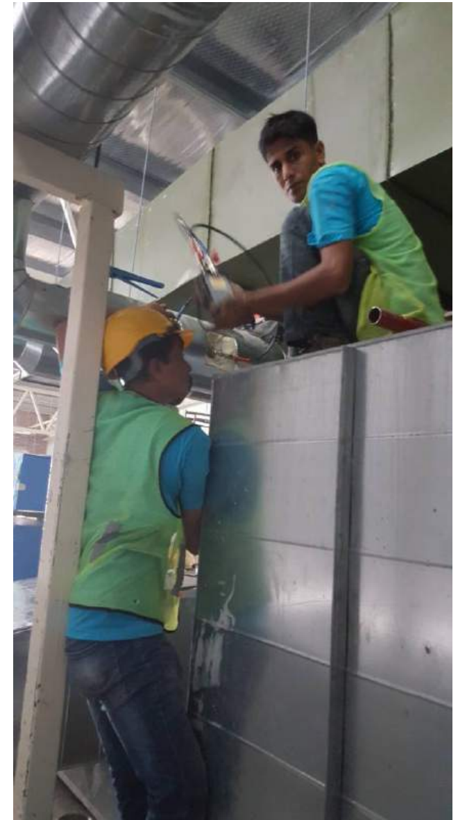
AHU/ FCU Water Balancing #3
