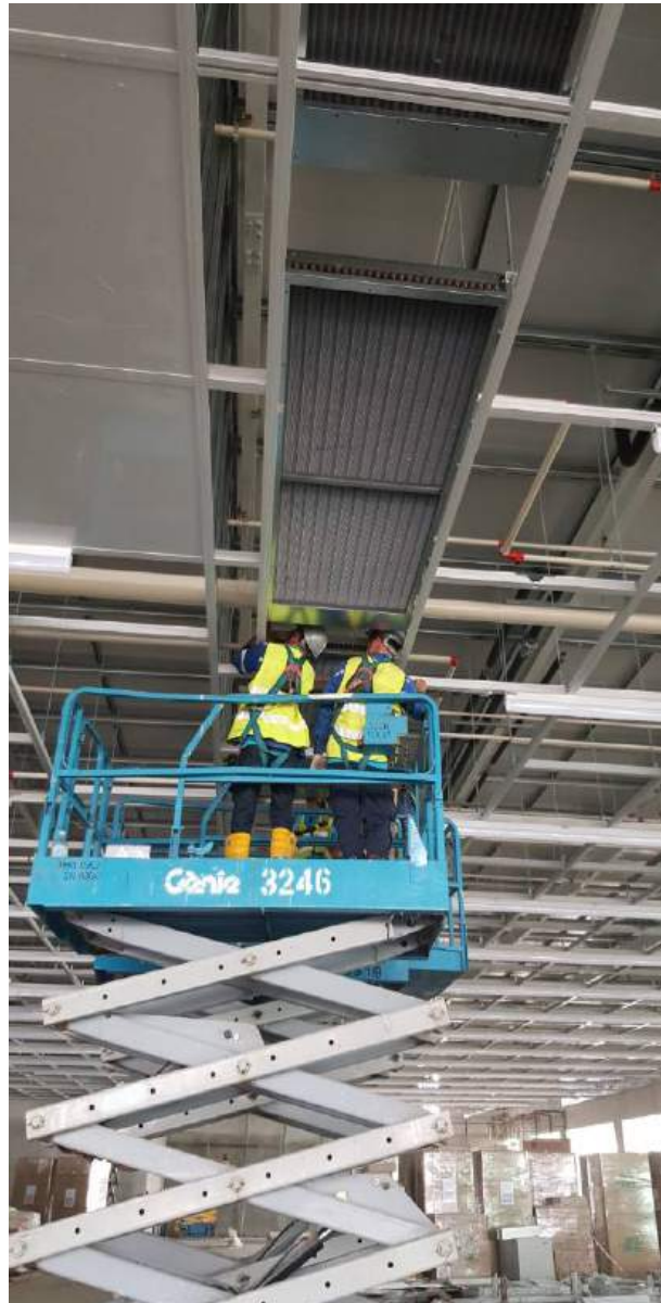
Dry Cooling Coil Installation #1
