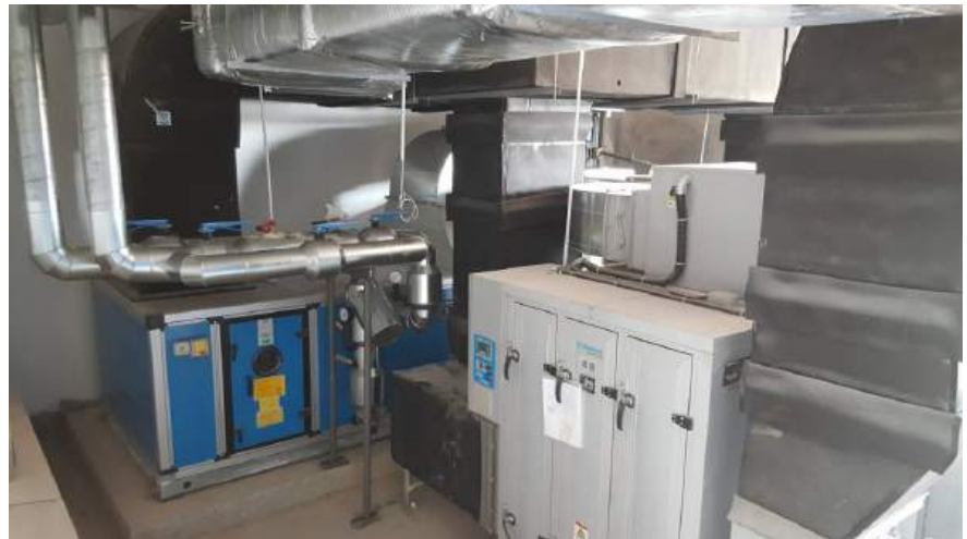
AHU & Desiccant Dehumidifier Installation
