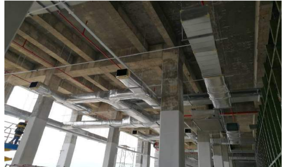
Ducting Installation #2
