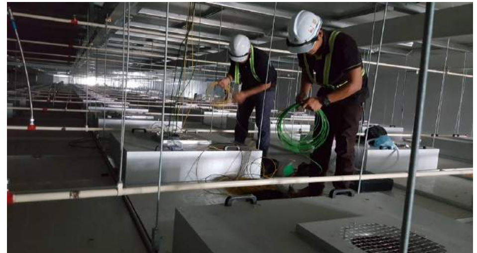
FFU Wiring Installation
