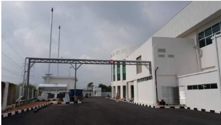
Steam Piping c/w Pipe Rack Installation
