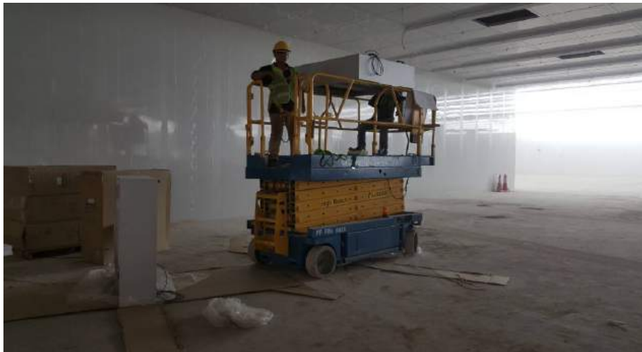
FFU installation Using Scissor Lift
