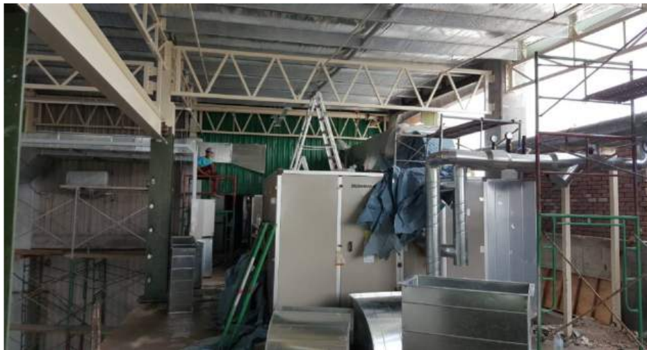
AHU piping & ducting installation
