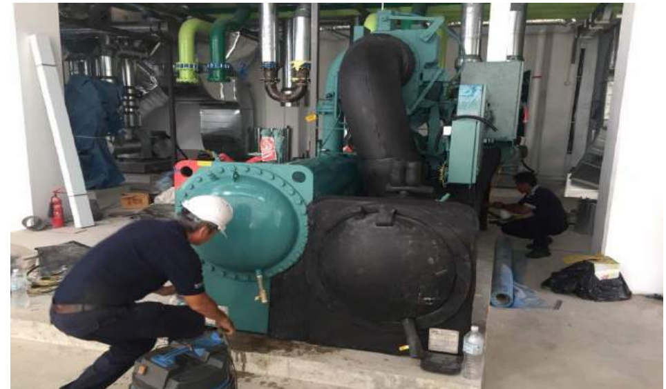
Chiller Final Positioning
