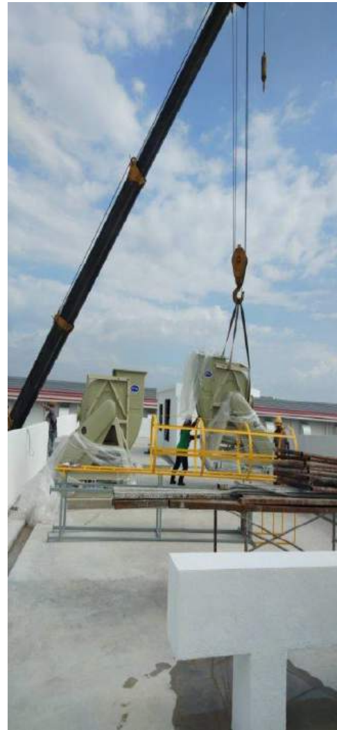
Scrubber Final Positioning
