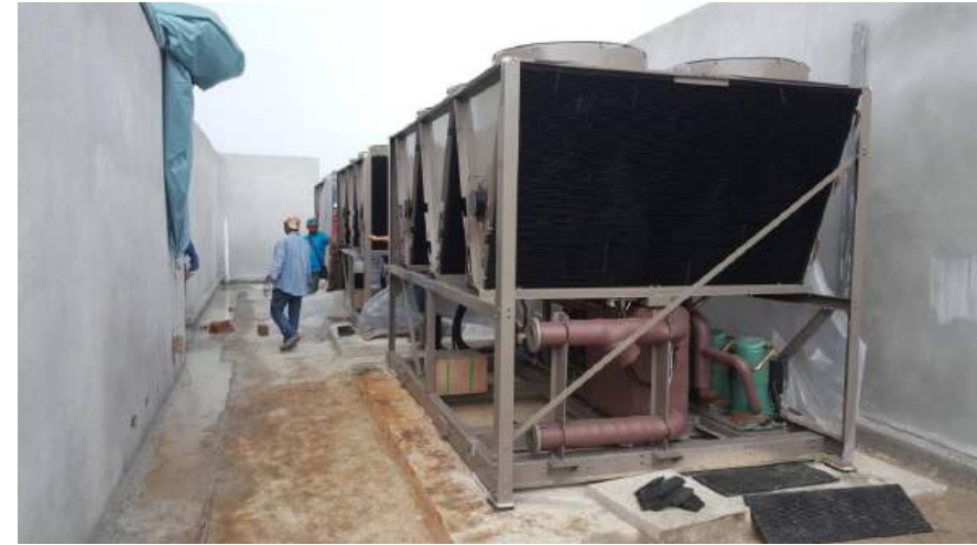
Chiller Final Positioning & Installation
