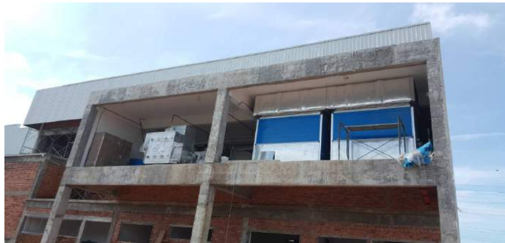
AHU, MCC & Ducting Installation
