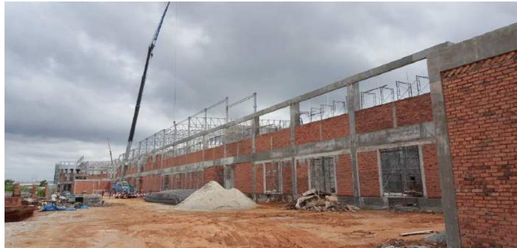
Air Compressor & AHU Hoisting
