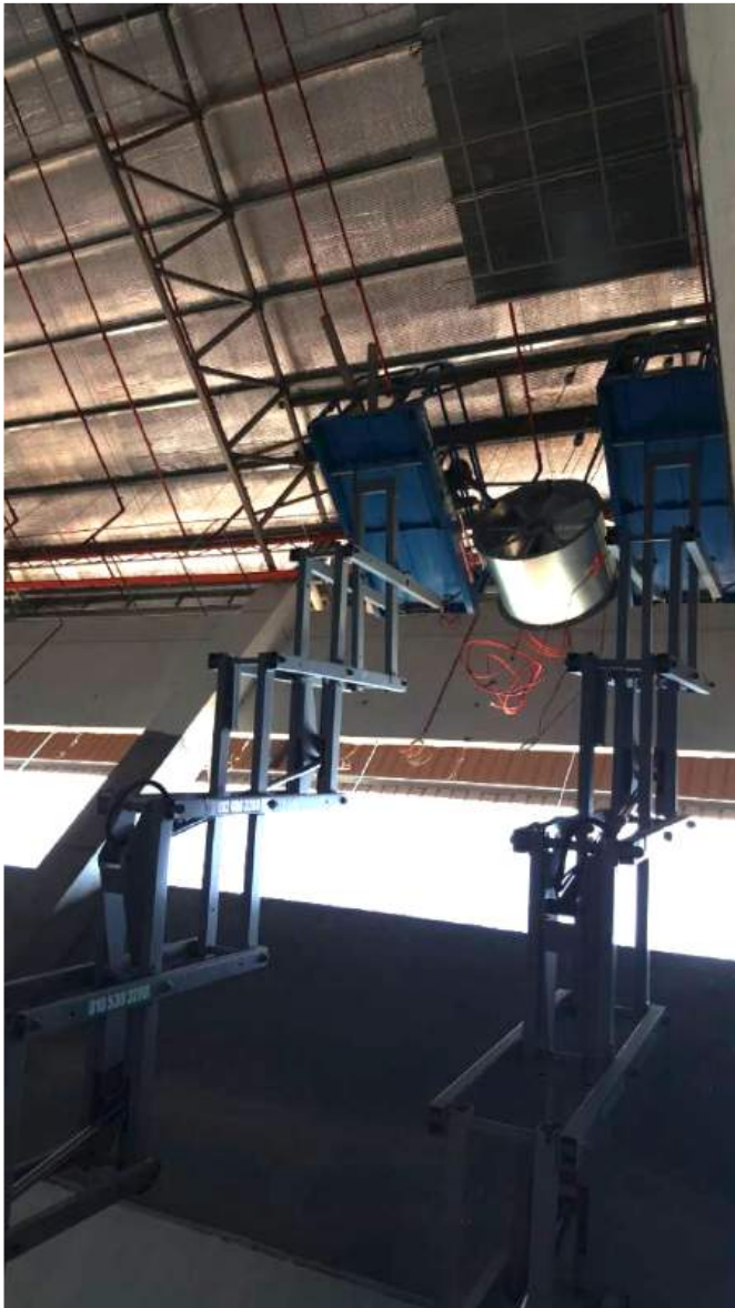
Smoke Spill Fan Installation
