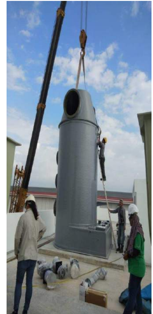
Silo Final Positioning
