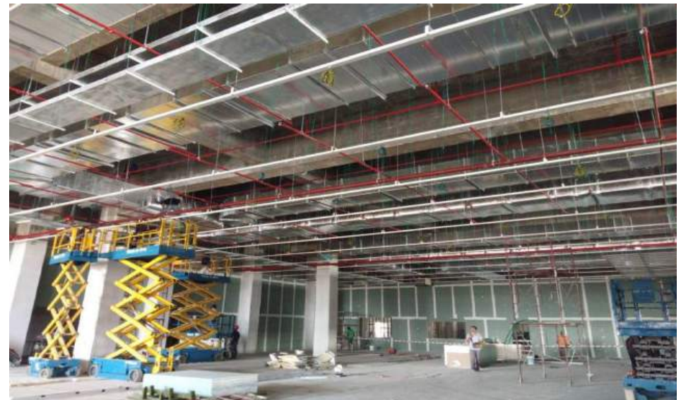
Ducting Installation #8
