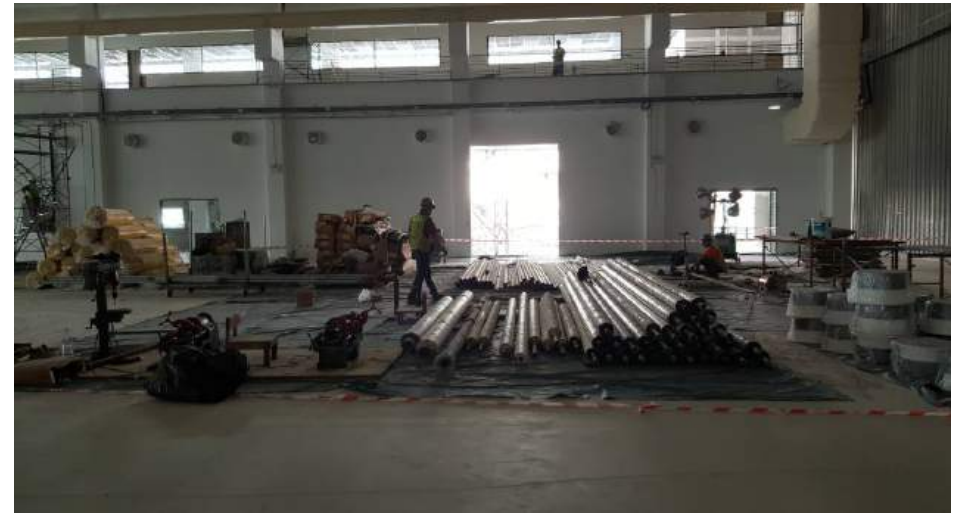
Chilled Water Piping On Site
