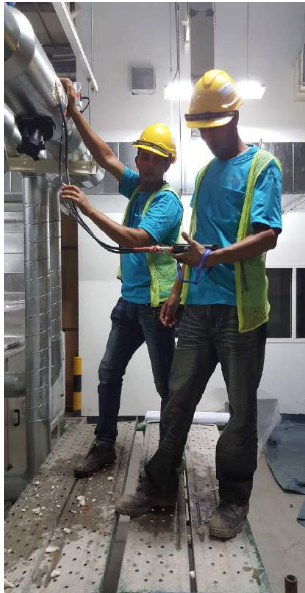
AHU/ FCU Water Balancing #2
