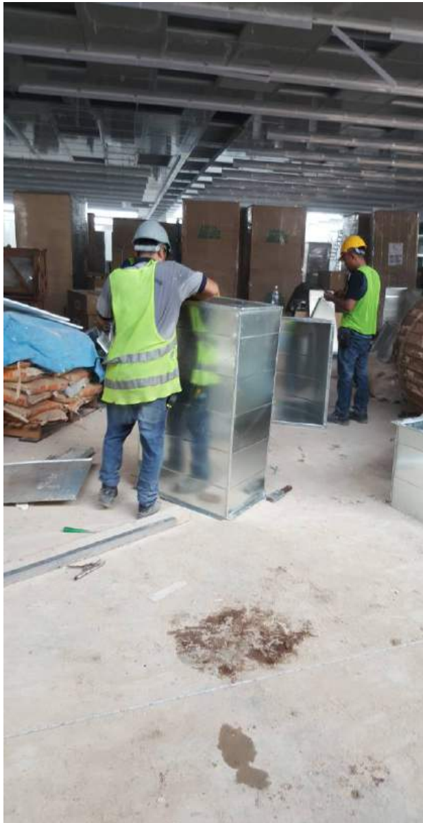
Ducting Installation
