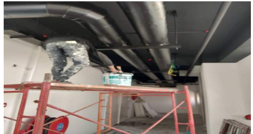
Exhaust Ducting Installation
