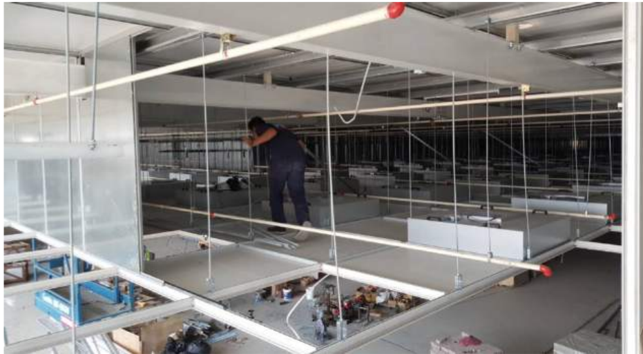
Walkable Ceiling c/w FFU Installation
