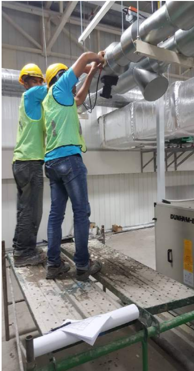
AHU/ FCU Water Balancing #1
